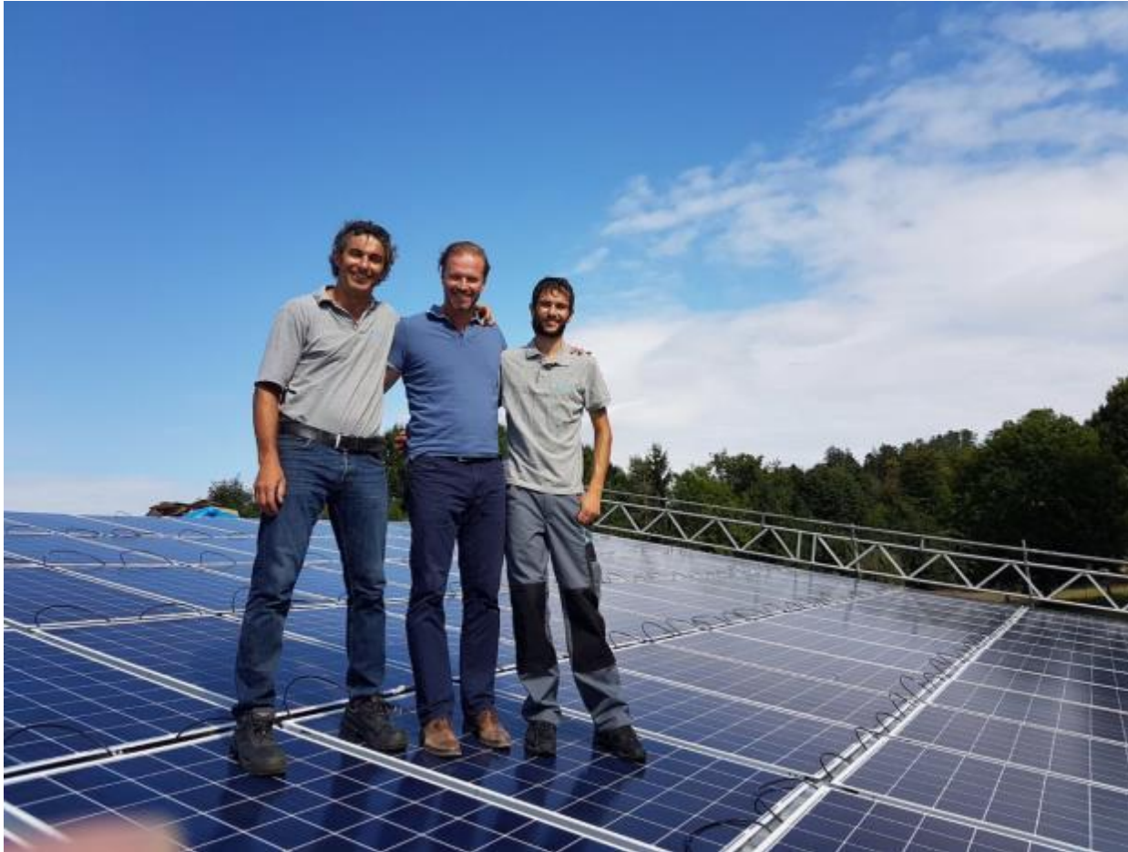
2000 sqm, 280 kWp, Bern - Production Hall – During installation
