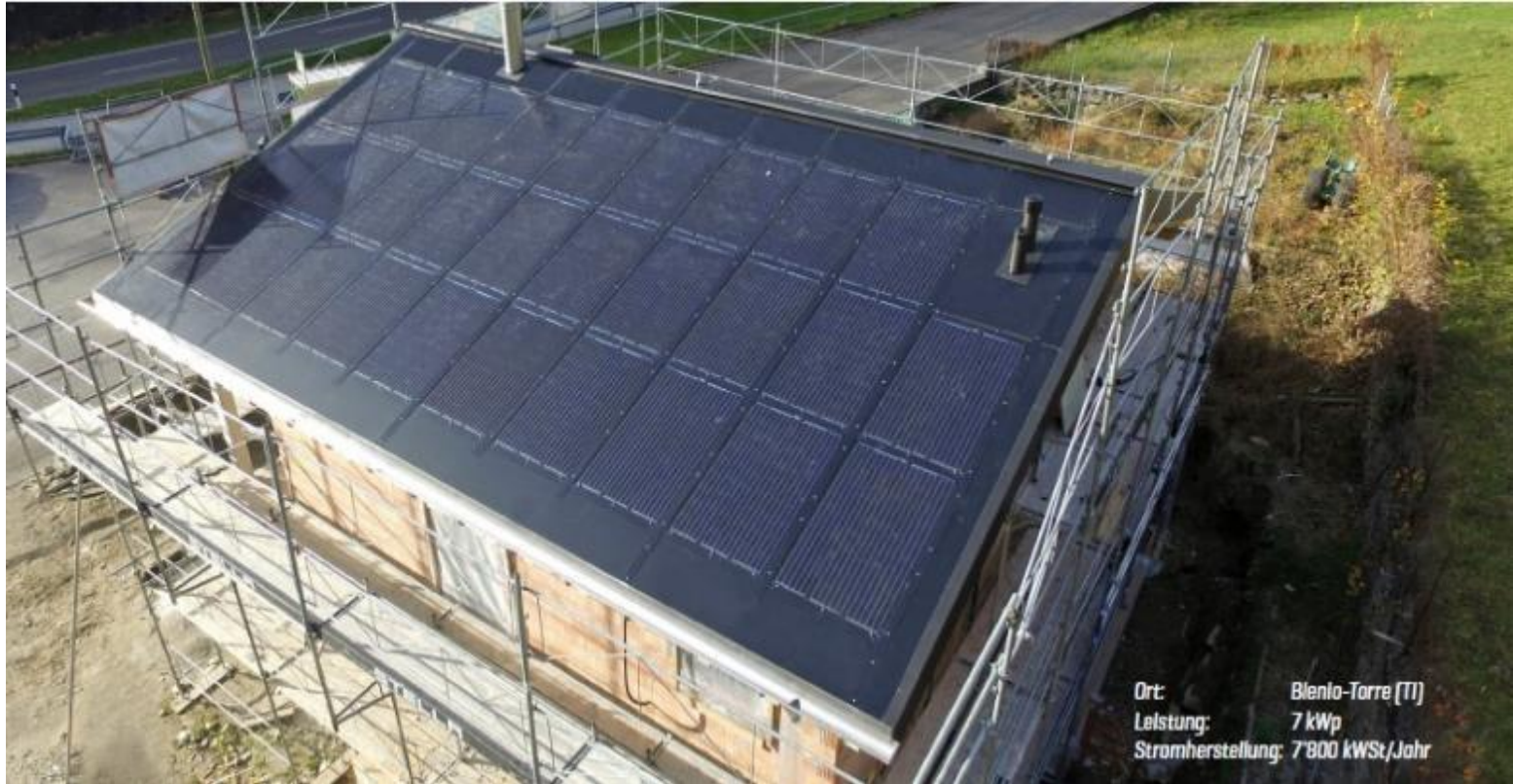
100 sqm, 7 kWp, Switzerland - Residential
